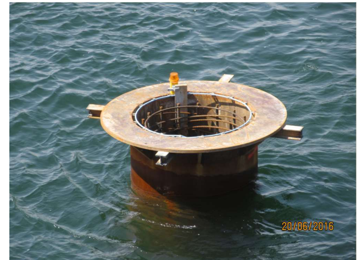
Soil excavation and placement of reinforcement cage
